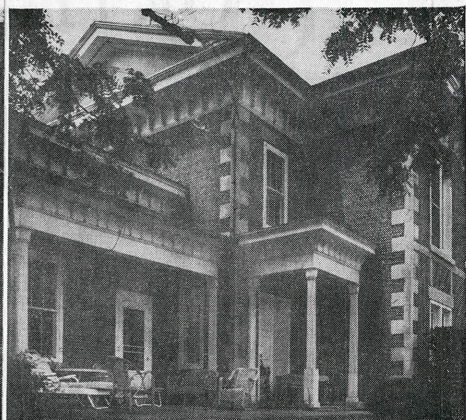
cobblestones, all of brown sandstone, were hauled by oxen from Lake Ontario beaches. The home was built in 1838 and claims a cobblestone smokehouse. At right is an 1844 cobblestone home on Rte. 14 in Yates County. The mansion's cobblestones were shipped by barge canal from Sodus Point on Lake
